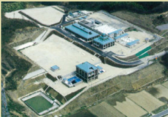
Arai Water Purification Plant (for Koriyama city)
